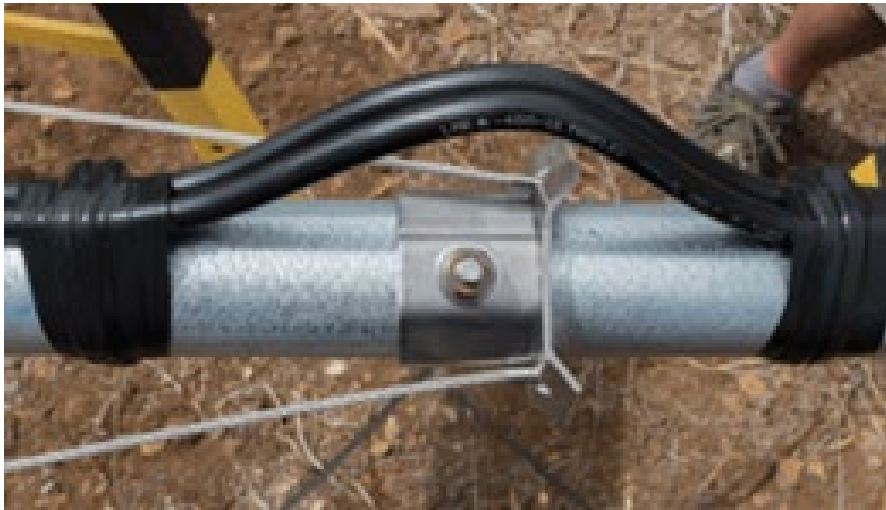
Figure 9—Coaxial cable fed around guy bracket
