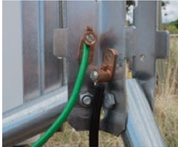
Figure 18—Earth connection
