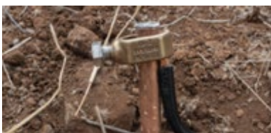
Figure 17—Earth connection
