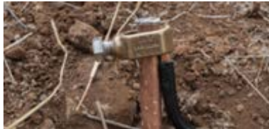
Figure 17—Earth connection
